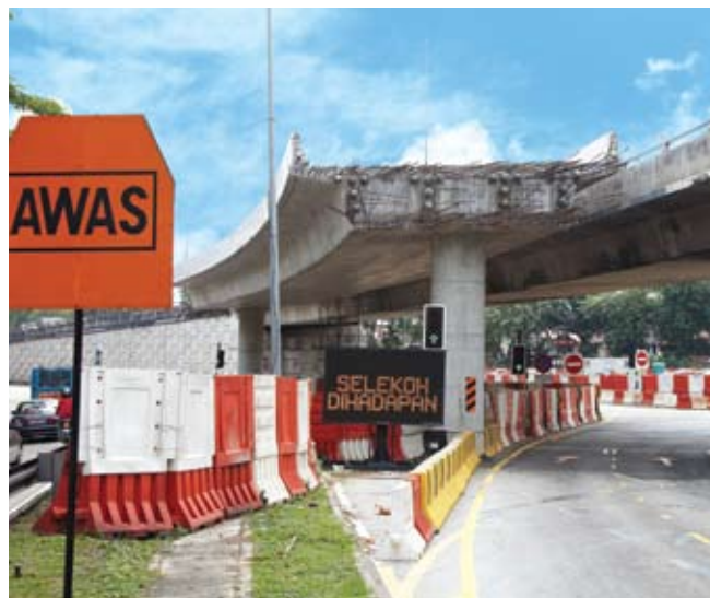
TTDI interchange upgrading works in progress.
